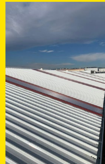
Moving forward on the green electricity transition
